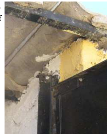
south door roof
