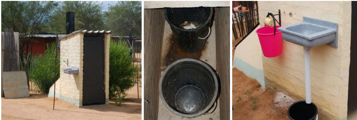
Fig. 2: Left: Otji toilet in Omaruru; Middle: Perforated faecal containers in the vault; Right: Basic handwash basin attached to the toilets. The pink bucket provides fresh water, the cup is used to fill the basin and the black bucket collects the greywater which can be used for irrigation (photos: F. Kleemann, GIZ, 2011).
